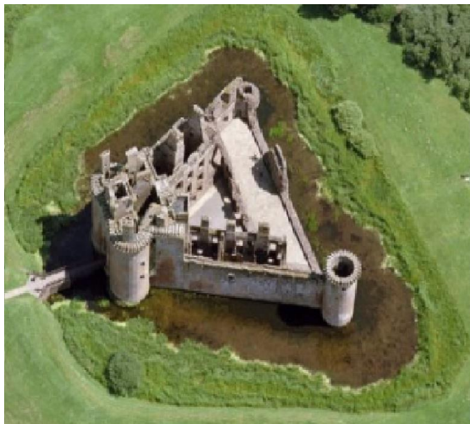
Figure 25: Caerlaverock Castle aerial view from NNW © HES SC1156766
