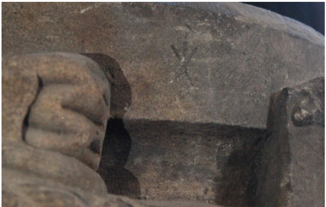
Figure 50: Glasgow Cathedral, mason's mark cut into the vertical face of a carved mould on display in Glasgow Cathedral © Lisa Craig Photography
