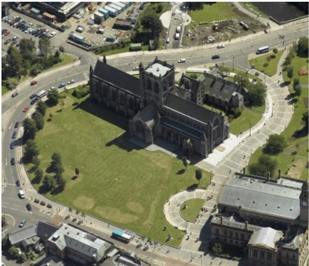
Figure 67: Paisley Abbey aerial view from NW © Canmore DP032412.
