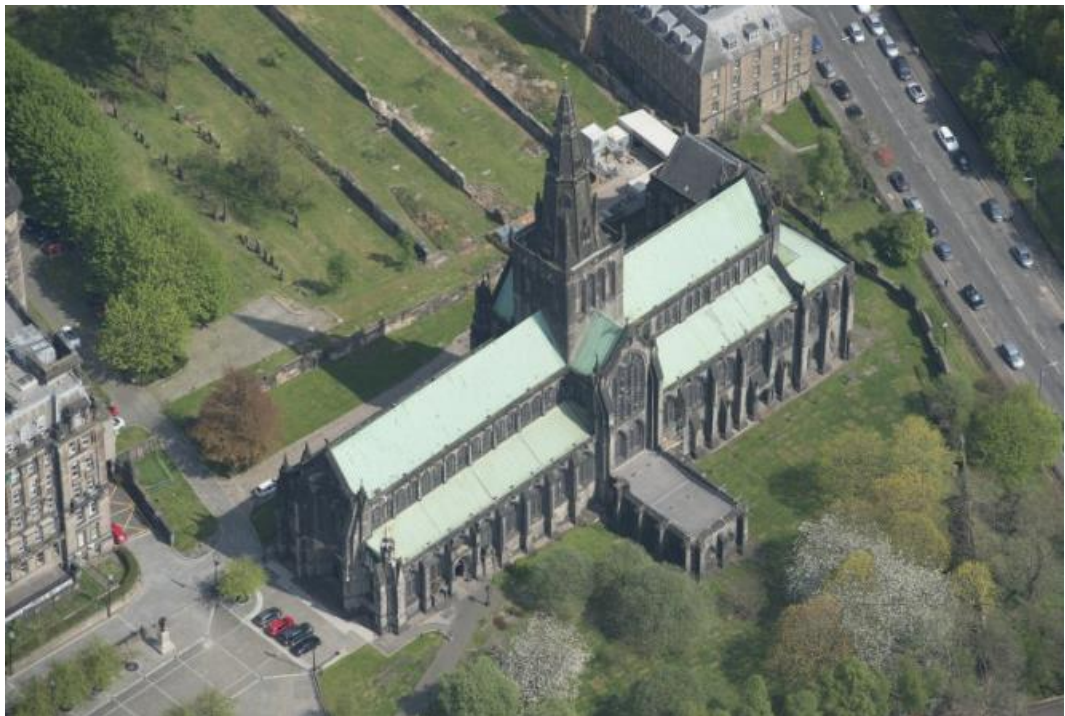
Figure 42: Glasgow Cathedral from SW © HES DP 234645
