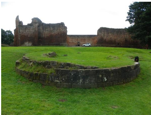
Figure 19: Foundations of NW tower at Bothwell Castle © Lisa Craig Photography
